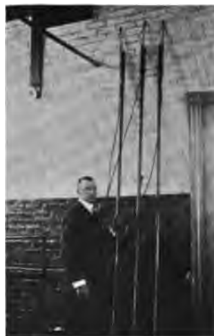
Fig. 9. Grounding Sticks for Station Service.
